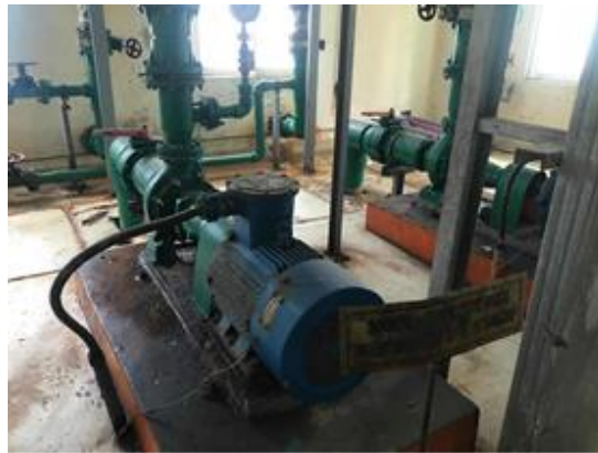
Gambar 8. Shock Dosing Pump
