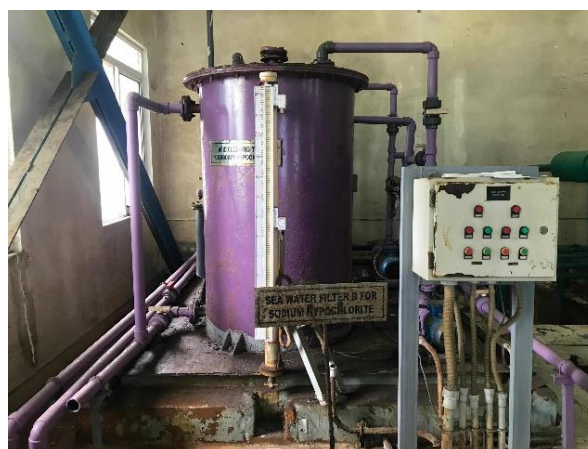
Gambar 3. Sea Water Tank Sodium Hypochlorite
