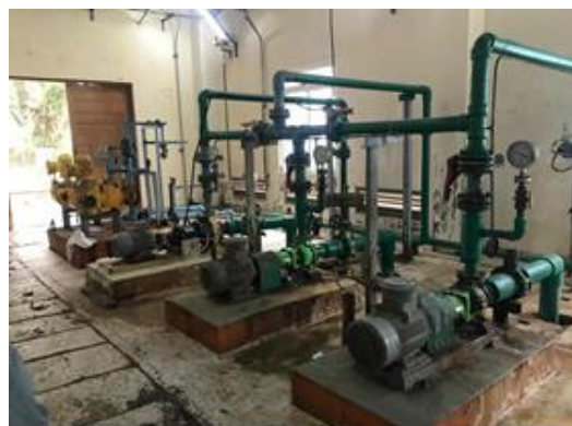
Gambar 7. Continous Dosing Pump
